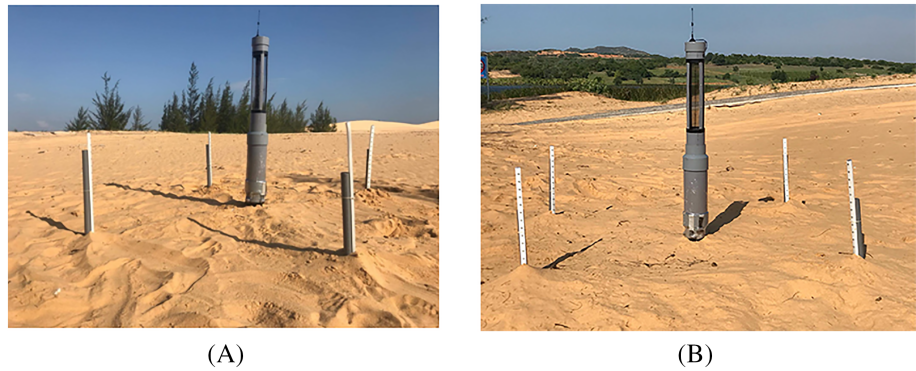
FIGURE 9 Prototype of the sensor structure installed in a real environment in Binh Thuan province, Vietnam
