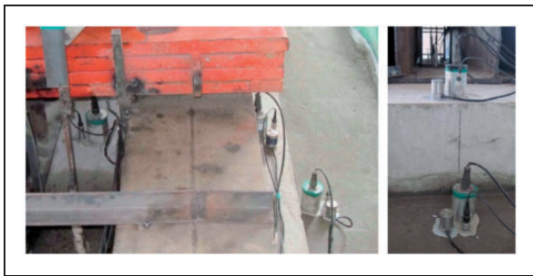
Figure 7. Installation of the testing sensors in the full-scale model.
